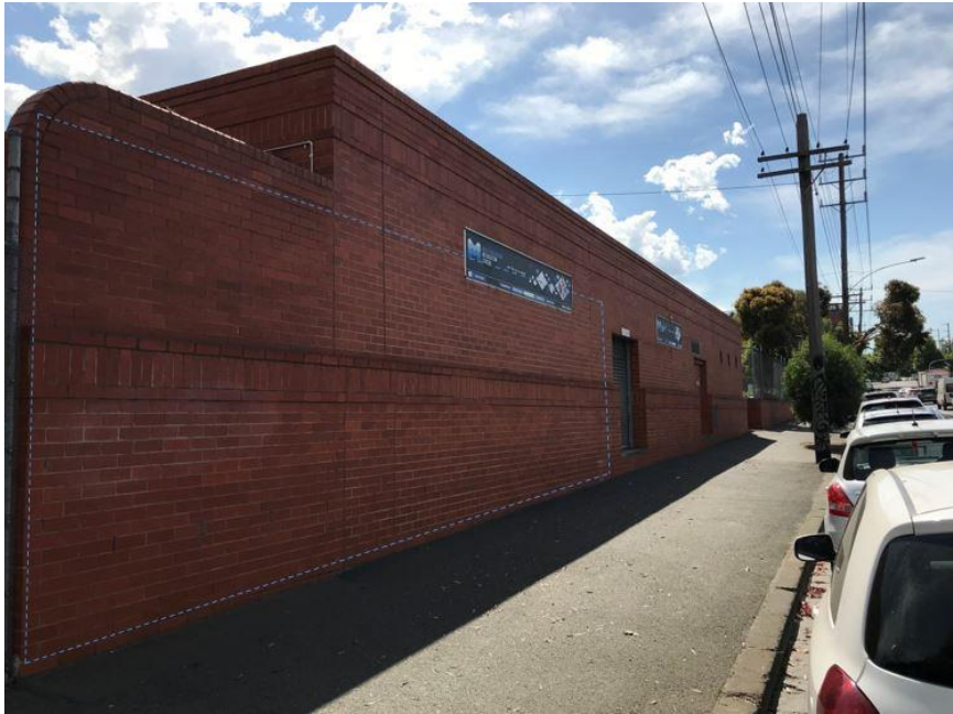
[External brick wall at North Melbourne Recreation Centre, approx. 10 x 3 metres]
